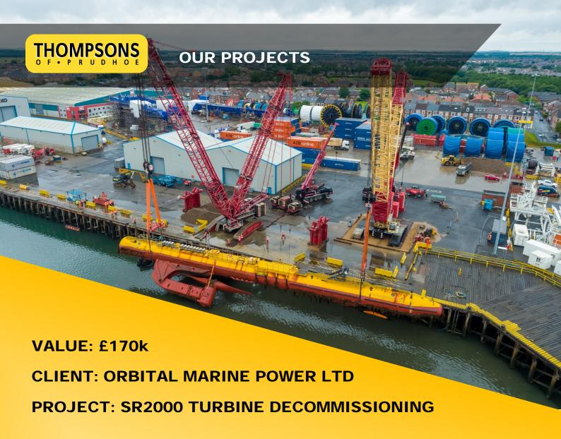
Thompsons of Prudhoe were contracted by Orbital Marine Power Ltd to undertake the safe decommissioning and waste disposal of a 2MW SR2000 Floating Tidal Turbine.
